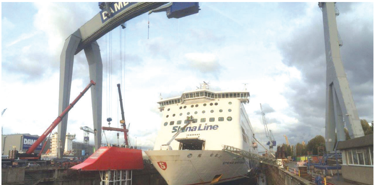
Image A5.8 Closed loop scrubbers installed on a Stena ship
