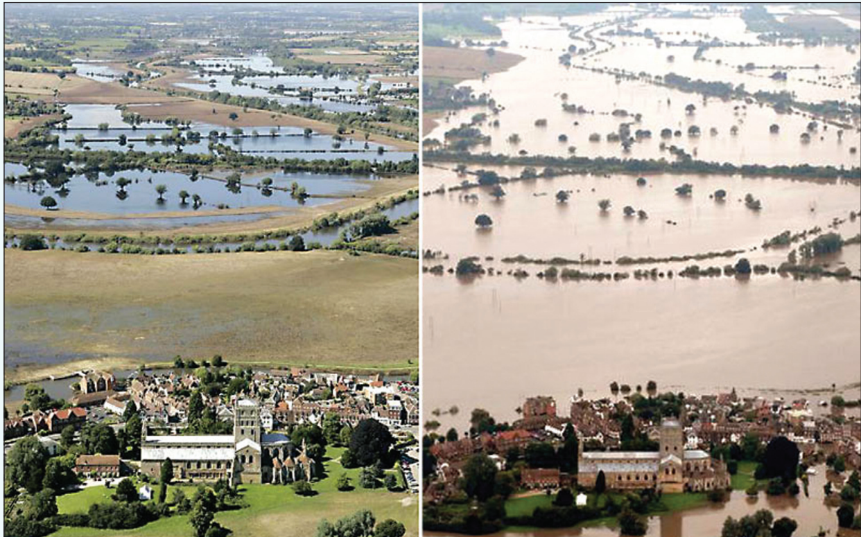
Flooding of a wastewater treatment works in Gloucestershire left 140 000 of the 160 000 homes it serves without piped water. Water supplies were restored to all properties within 10 days but were not safe to drink until 15 days after the flood. Since this event, 1000 m of semi-permanent flood barrier to a height of 13.5 m AOD (Above Ordnance Datum) has been installed to protect against future flooding (Environment Agency, 2010a).
