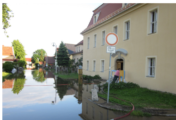
Flooded street in the Brockwitz district, 2013 © Coswig City
