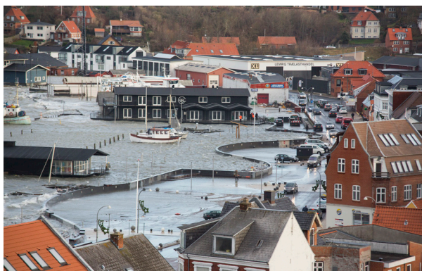
'Le Mur' protecting Lemvig harbour © Mads Krabbe
